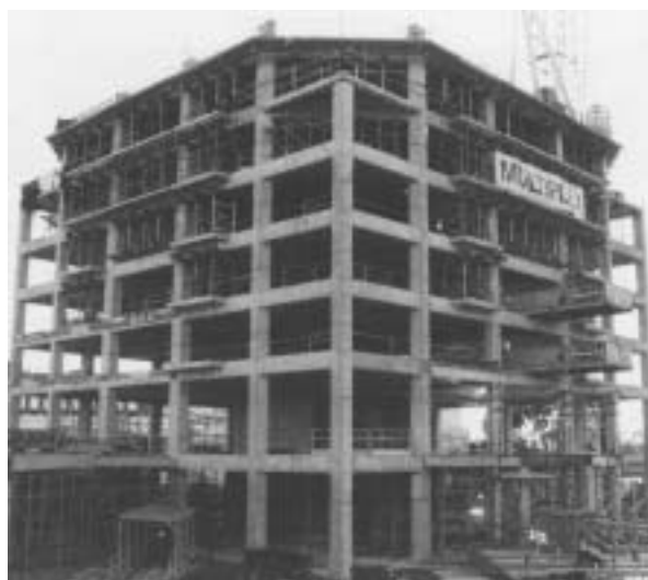
Spencer on Byron building under construction
