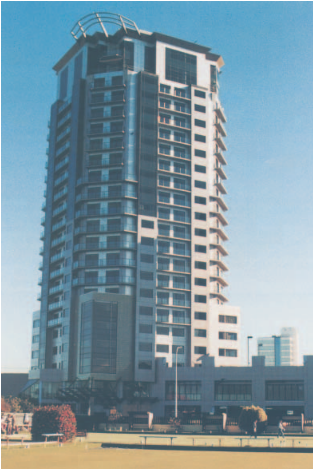
Spencer on Byron completed structure
